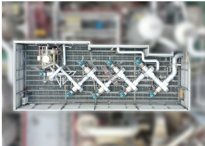
Vapor Compression Heat Pump Technology: Vapor Compression with serial connection of eight VapoFlex
