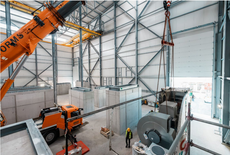
Image caption: Machines being positioned on the prepared concrete blocks.
