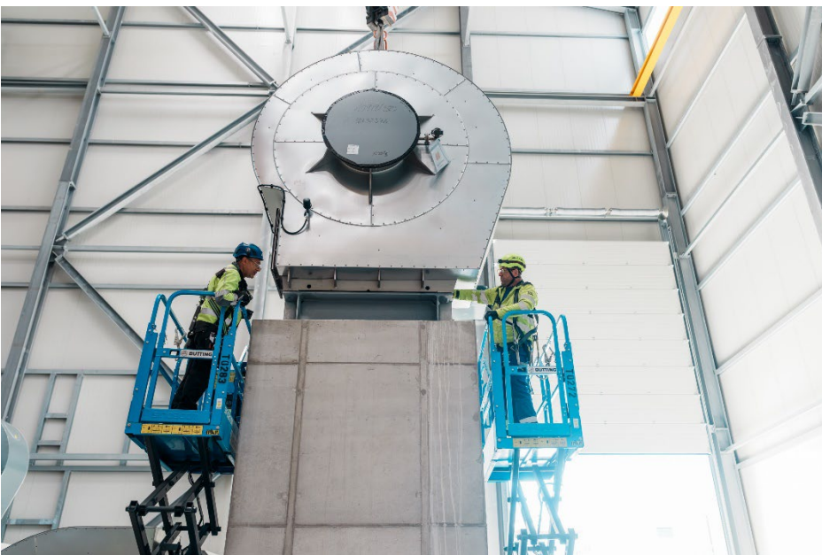
Image caption: Preliminary installation and securing of the units at BASF.
