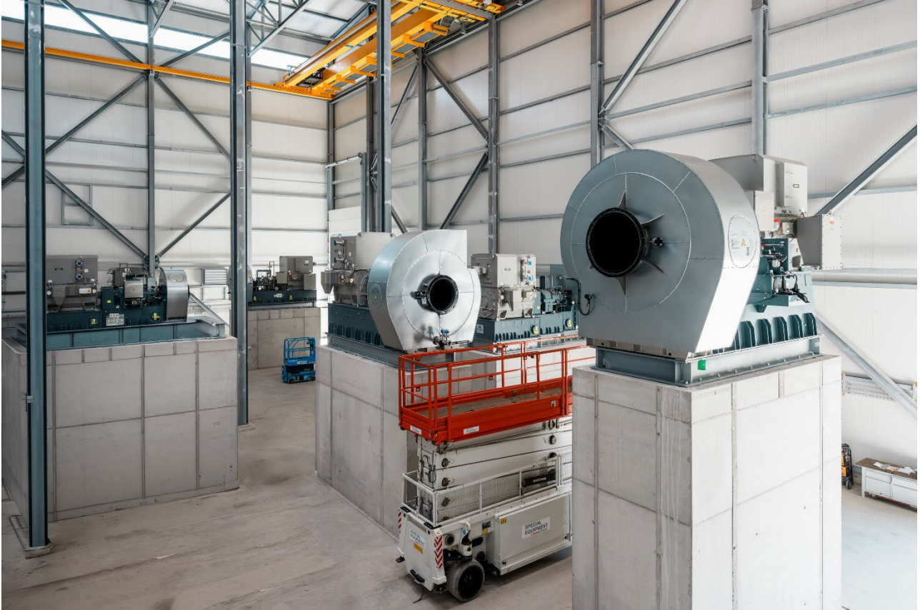
Image caption: The first PILLER compressors have been successfully positioned: With the machines now placed on their designated concrete bases, another key milestone in the major BASF project has been reached.
